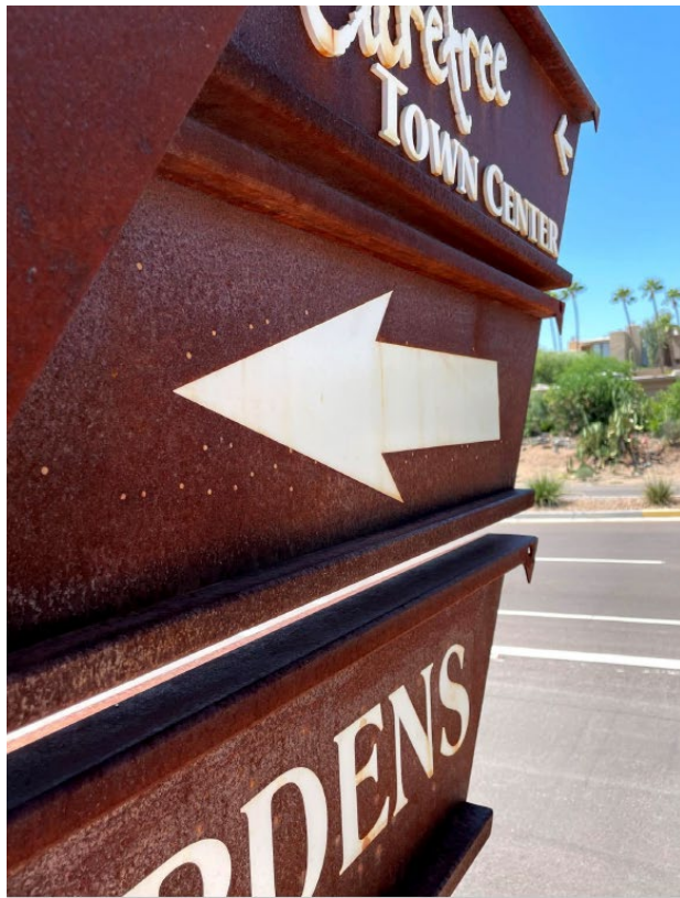
Metal with Rusted Finish
