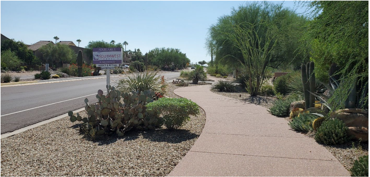
Existing Section of Sidewalk Along Cave Creek Road
