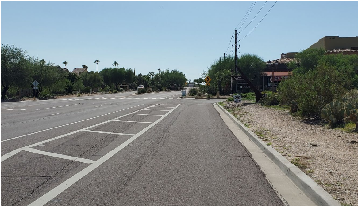
Existing Turn Lane on Cave Creek Road
