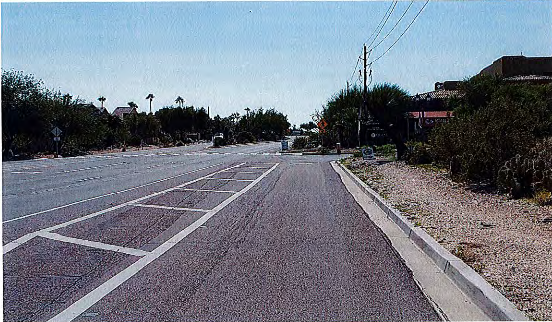
Existing Turn Lane on Cave Creek Road
