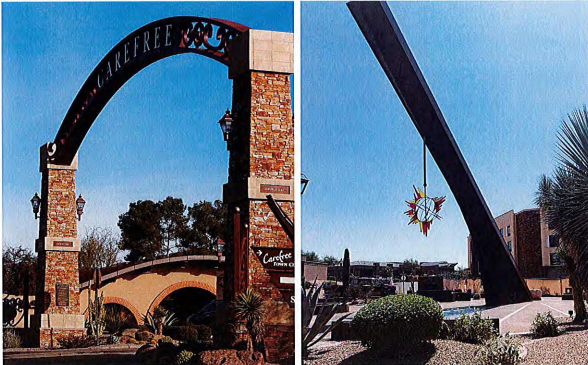
Existing Gateway Signage
