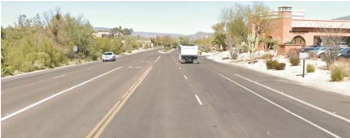
Figure 3: Tom Darlington Drive near Carefree Marketplace (Looking Northbound) Source: Google Earth (2021)
