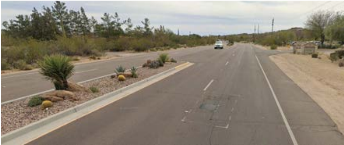
Figure 13: Cave Creek Road near Elbow Bend (Looking Southbound) Source: Google Earth (2021)
