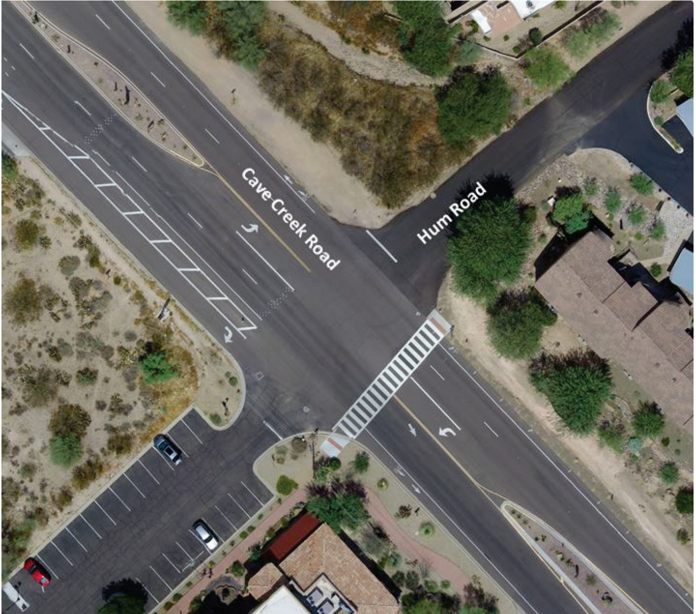
Figure 4: Cave Creek Road and Hum Road intersection
