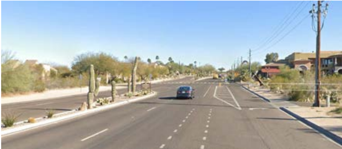
Figure 17: Cave Creek Road near Hum Road (Looking Southbound) Source: Google Earth (2021)
