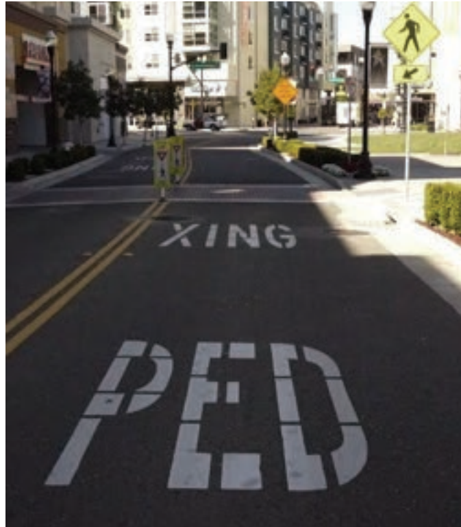
Figure 29: Pedestrian Crossing Ahead Pavement Marking
