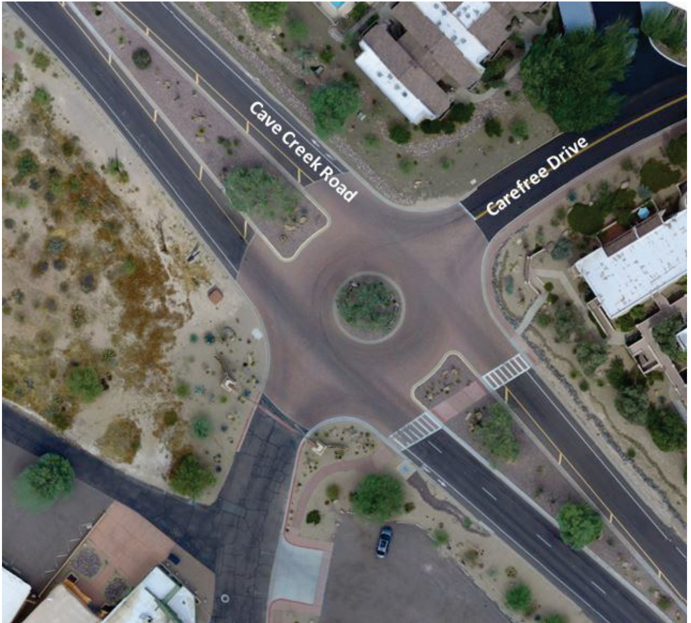
Figure 5: Cave Creek Road and Carefree Drive Intersection
