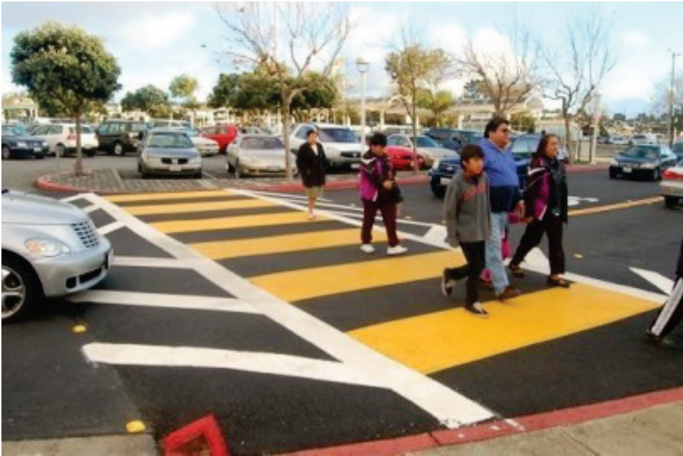
Figure 20: Raised Pedestrian Crosswalk
