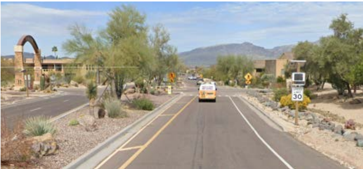
Figure 14: Cave Creek Road near Carefree Drive (Looking Northbound) Source: Google Earth (2021)
